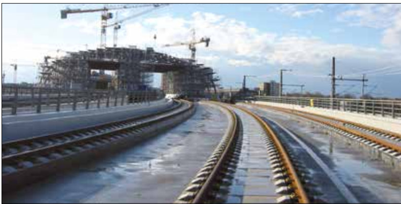
Hauptbahnhof, Berlin Central Railway Station, Berlin
